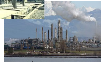
Examples of Energy Infrastructure
