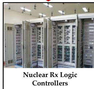
Nuclear Power Plant Digital Control System
